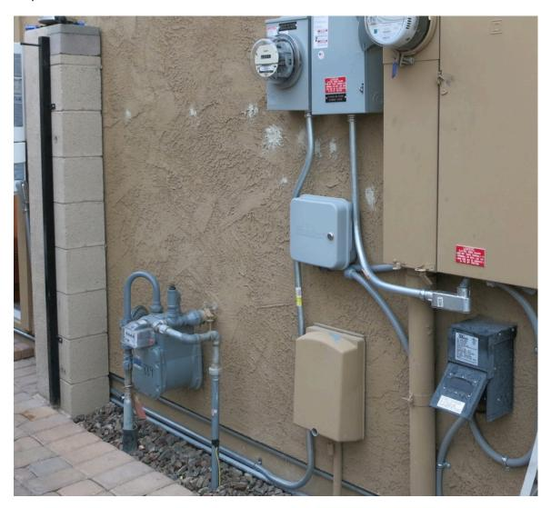
7. Contractor did not install wire to match permit specification. Permit called for 2AWG between the combiner box and contractor installed 6AWG. Permit also called for 4AWG between the inverter and the SES and contractor installed 6AWG. This was one of the main points of why the project failed city inspection.
