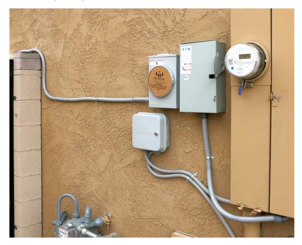
6. I advised the contractor that the plastic liquid tight conduit is not acceptable, both per the permit and aesthetically. The contractor replaced the plastic conduit with EMT, however the incorrect size was again used and did not match the specifications of the permit. This was one of the main points of why the project failed city inspection.
